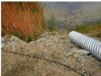
Photo 10: Closer view of POND1 outflow pipe outlet (OUT1) set on rip-rap into POND2.
