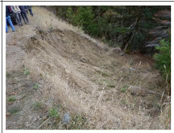
Photo 38: Image of landslide (SLIDE2) downgradient of the road located between stream crossing C2 and POND1 caused by road development, grading and surface runoff.
